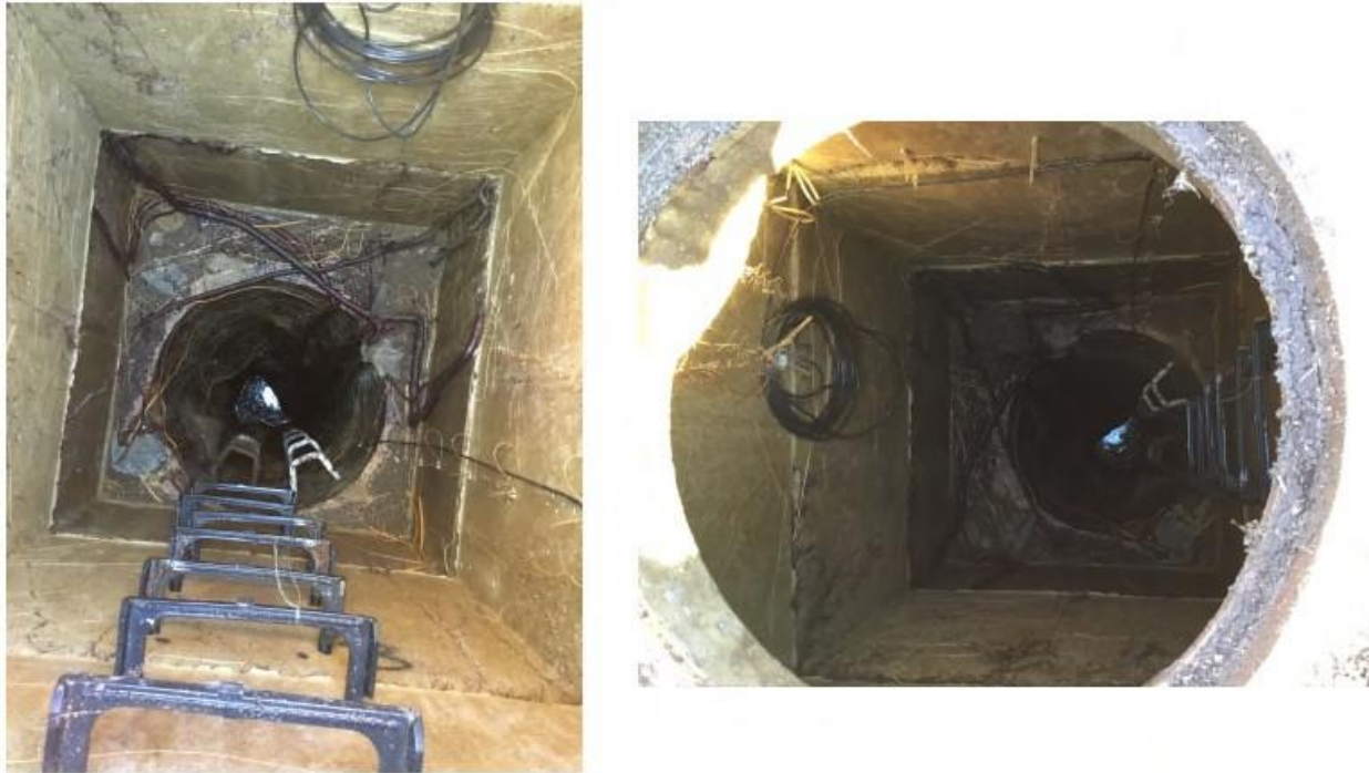
Figure 3-1: Downhole Photos of MH-4
